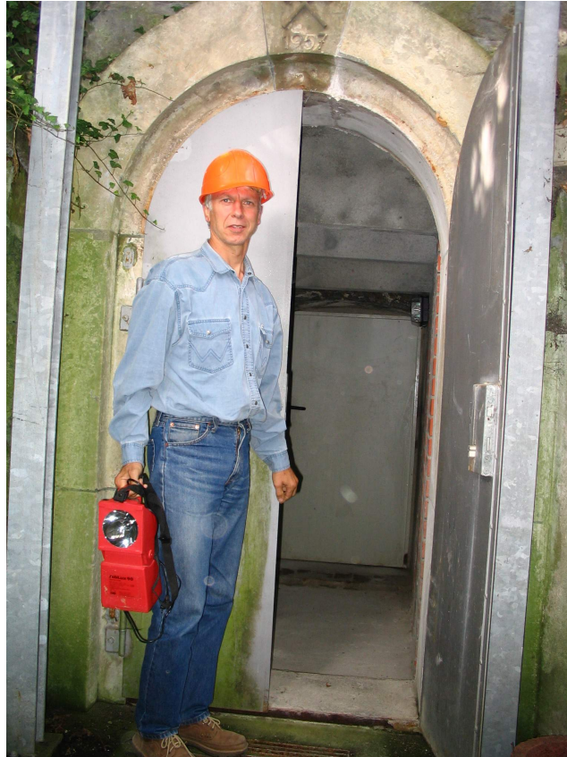
Figure 5.21: Entry to mining tunnel.
